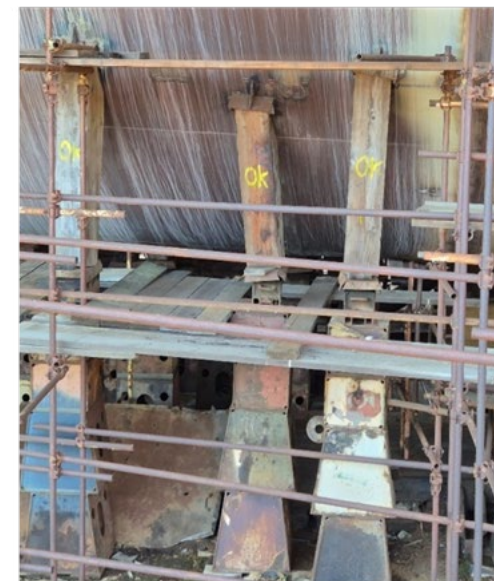
Pomaci upornih elemenata uslijed zastoja gradnje / Shift of support blocks under the vessel due to an extended construction downtime
